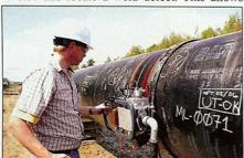
pipeline contractors to implement engineering methods to assess the strength of a weld, saving potential rework costs that could ultimately affect the weld's integrity. It uses ultrasonic technology as opposed to radiography, making inspection possible immediately following the welding process. 978-437-1410, www.ge.com.
