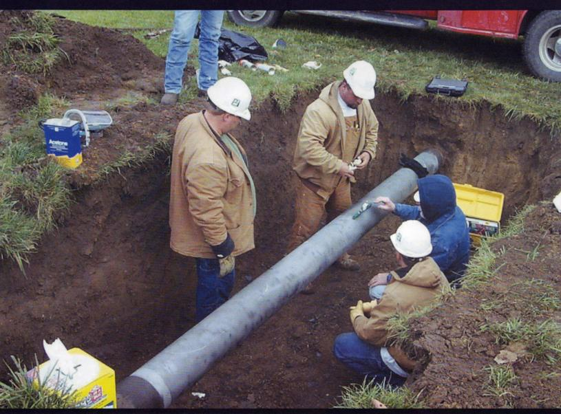
Assisting technicians in the field to measure the amount of corrosion on a section of pipe accurately and with 1/1000 of an inch
